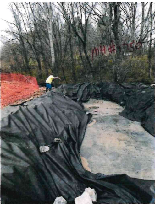
Adding New Filter Fabric
