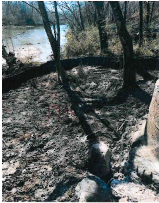
Spread with Enzyme and Lime
