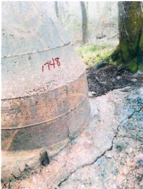
Wash Down and Cleanup Around 1748
