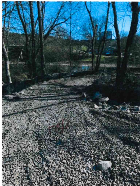
New Silt Fencing
